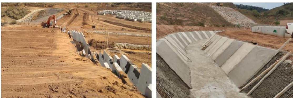
Figura 5 - Descida d'água (talude OE) e canal CP07(Platô)
