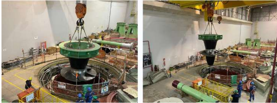
Figura 15 – Rotor Kaplan
