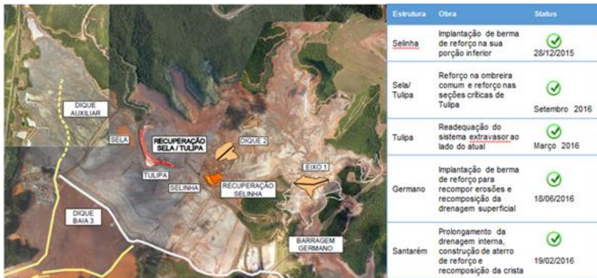
Figure 8 : Emergency works of containment and stabilization executed during the rainy period 2015/2016
