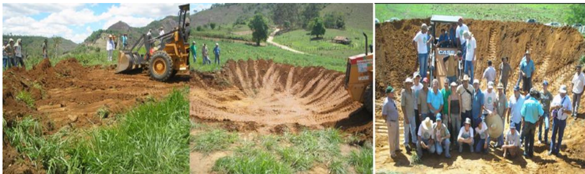
Figure 62: Construction of catchment basins (archive Instituto Terra).
