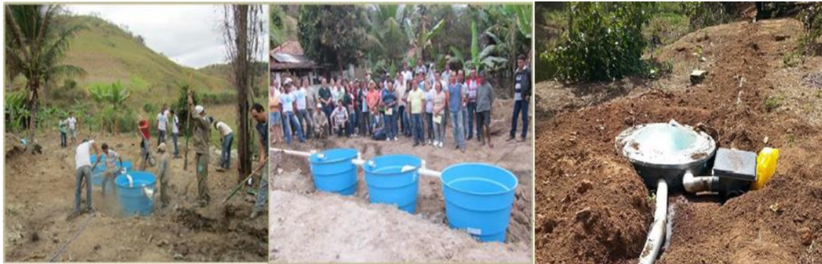
Figure 59: Installation of septic tanks (archive Instituto Terra).
