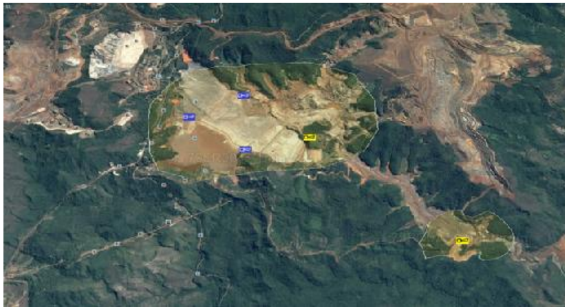
Figure 13: Sirens of the Germano and Santarém dams .
