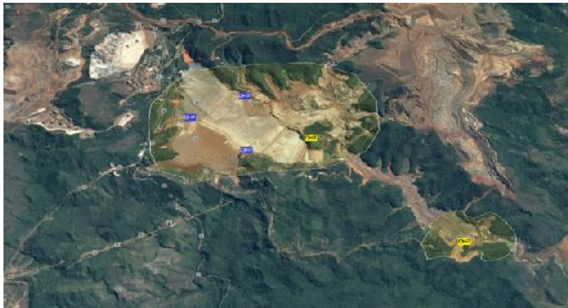
Figure 13: Sirens of the Germano and Santarém dams .
