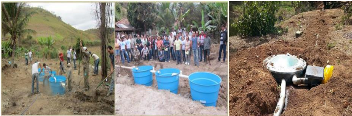
Figure 58: Installation of septic tanks (archive Instituto Terra).
