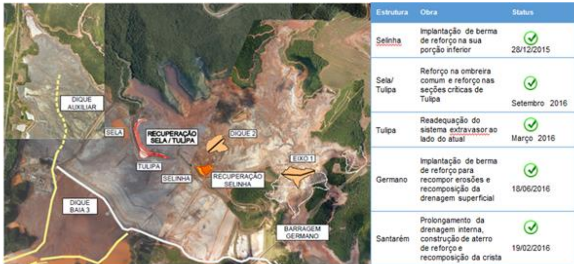
Figure 8 : Emergency works of containment and stabilization executed during the rainy period 2015/2016
