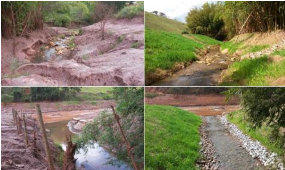
Figure 23: Environmental recovery of tributary TG51.
