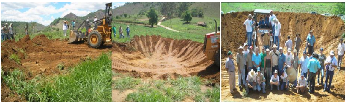
Figure 59: Construction of catchment basins (archive Instituto Terra).
