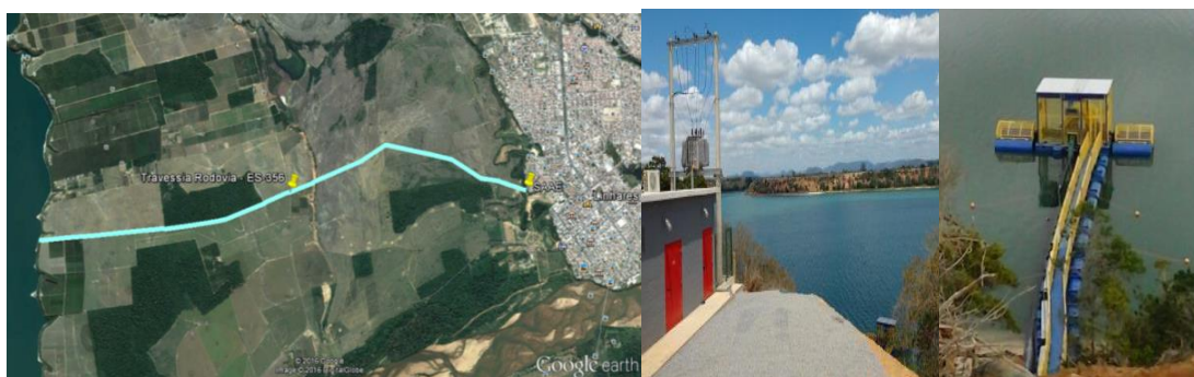
Figure 67: Aqueduct from Lagoa Nova in Linhares.
