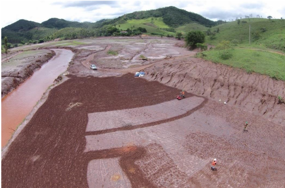
Figure 42: Preparation of the soil utilizing manual and semi-mechanized methods of scarification of the substrate, seeding and fertilization being executed near Paracatu de Baixo
