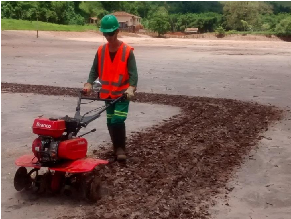
Figure 42: Semi-mechanized preparation of the substrate using a motor-cultivator near Barra Longa.
