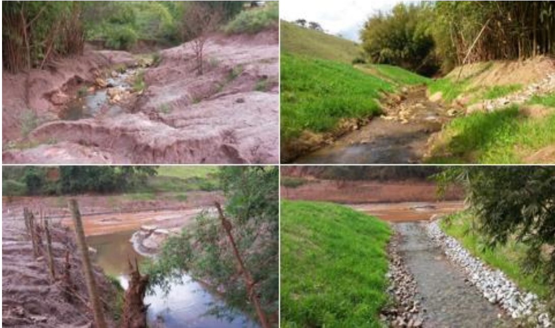
Figure 24: Environmental recovery of tributary TG51.
