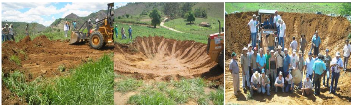
Figure 56: Construction of catchment basins (archive Instituto Terra).
