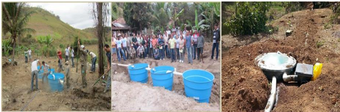
Figure 55: Installation of septic tanks (archive Instituto Terra).
