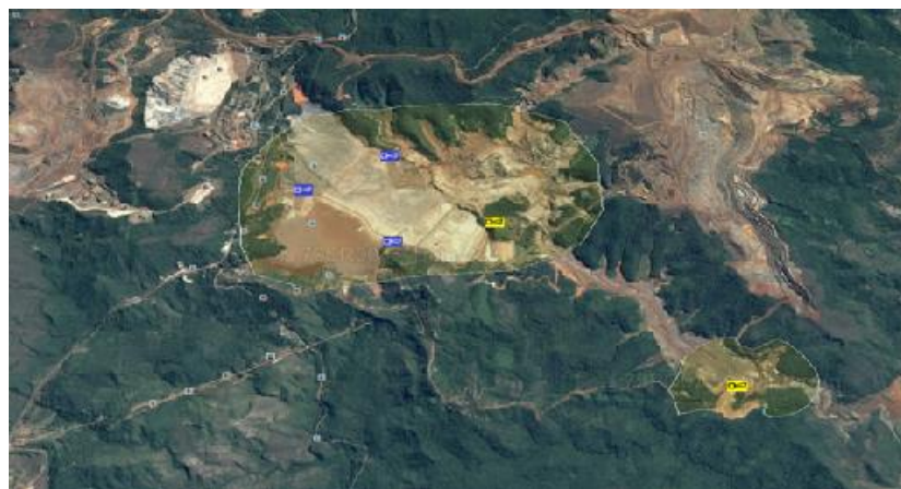
Figure 14: Sirens of the Germano and Santarém dams .
